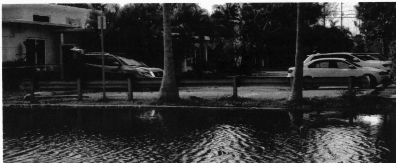
Miami Beach canal seawall nearly overtopped during king tide event. Source: Miami Beach
