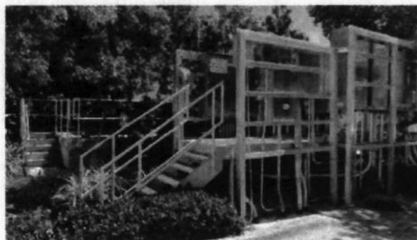
Elevated stormwater pump station and electrical panels. Source: Miami Beach
