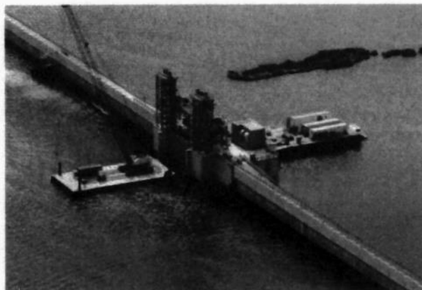
Lake Borgne Surge Barrier gate. Source: U.S. Army Corps of Engineers
