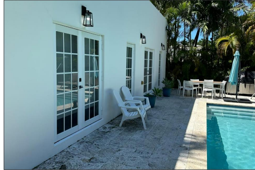
Figure 1A. View of existing openings on the back of the property.
