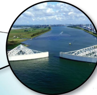
Surge Barrier Gates
