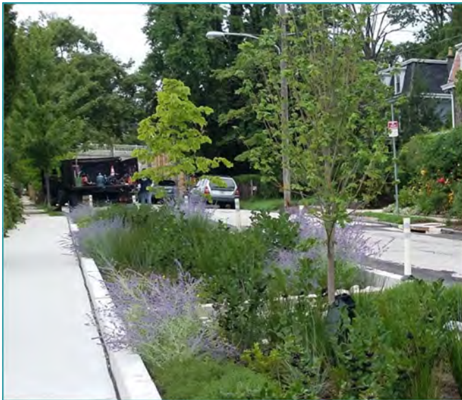
Stormwater planters in public right-of-way
