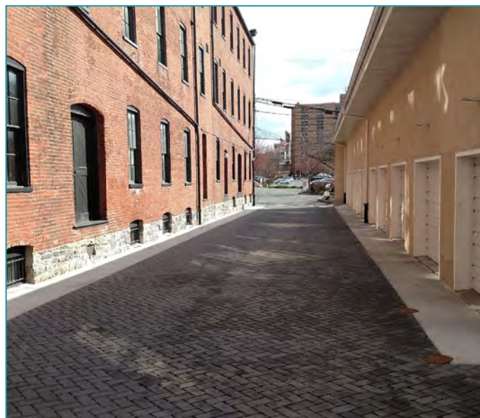
Permeable pavers above an infiltration trench in an urban alley
