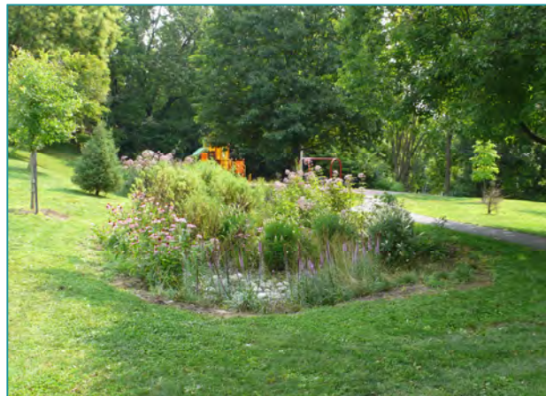
Bioretention facility near the entrance to a public park
