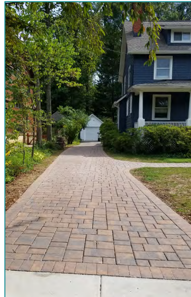
Permeable pavement driveway
