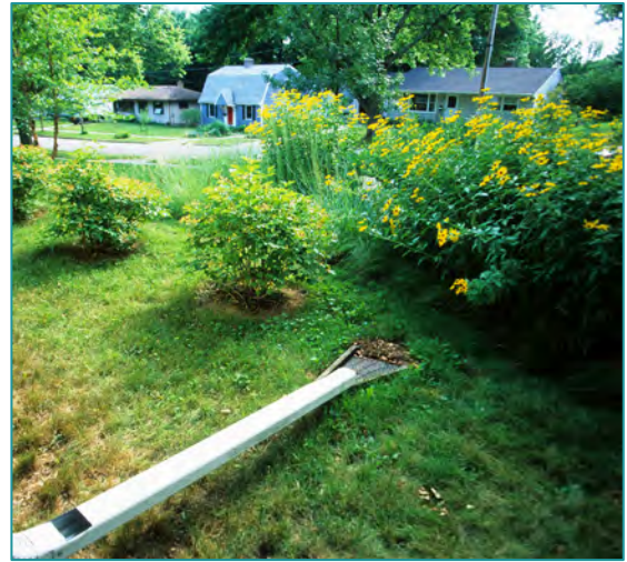
Downspout that has been disconnected from a stormwater pipe and directed toward landscaped area (Source: Wisconsin Department of Natural Resources)
