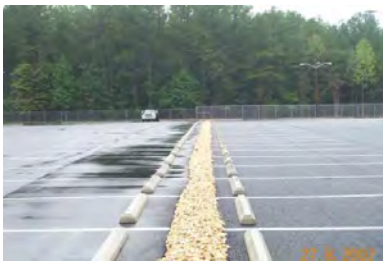
Normal (left) and Porous Asphalt (Right)
