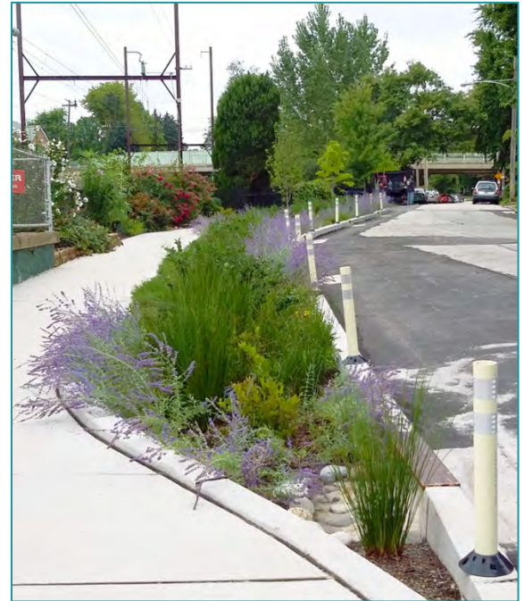
Stormwater planter between a road and newly constructed sidewalk
