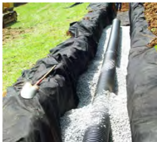
Infiltration Trench
