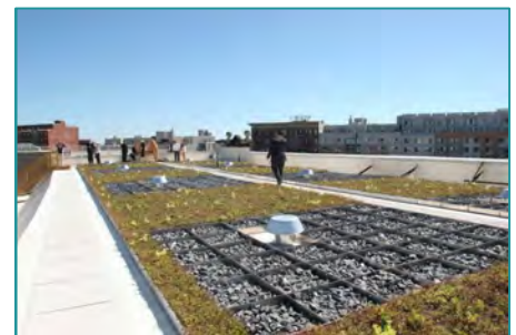
Example of a building with sections of both blue and green roof systems (Source: NYC Environmental Protection)
