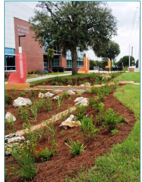
Bioretention facility at the University of Florida Southwest Recreation Center (Source: Stephen Hofstetter, Alachua Co. Env. Protection Dept.)
