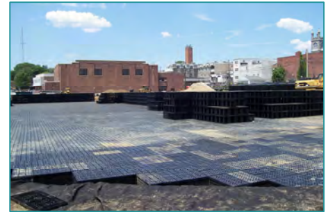
Subsurface infiltration/storage system with plastic chambers being installed along with the raising of a playfield at a school
