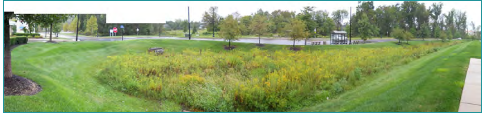
Detention basin planted with dense native vegetation and designed for infiltration
