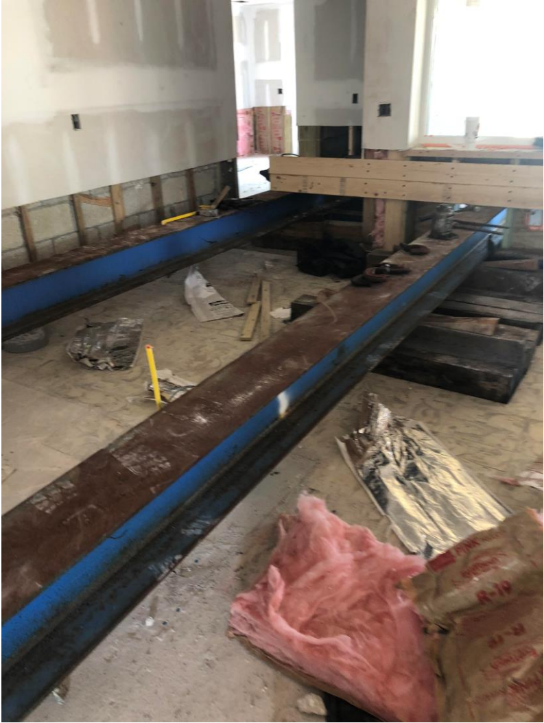
Rigging the home for elevation, building the steel interior frame
