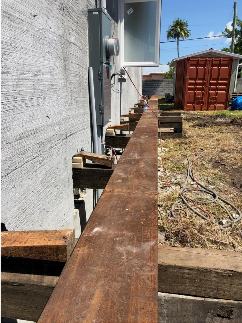
Rigging the home for elevation, building the steel interior frame
