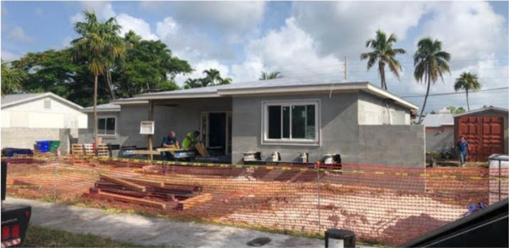
Rigging the home for elevation, building the steel interior frame
