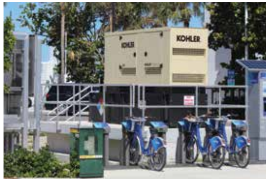
Pumps and generators installed in the Sunset Harbour neighborhood are a visible part of the city's stormwater strategy.
