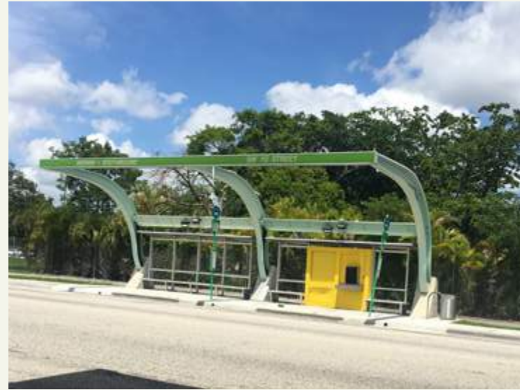
South Dade Transitway Stop. The SMART Plan intends to advance six of the PTP's rapid transit corridors, along with a network system of Bus Express Rapid Transit (BERT) service, in order to implement mass transit projects in the county.
