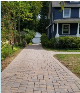
Permeable Paver Driveway Source: Jacobs
