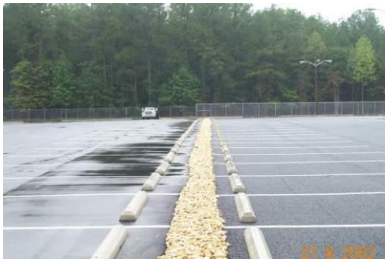
Normal (left) and Porous Asphalt (Right) Source: Jacobs
