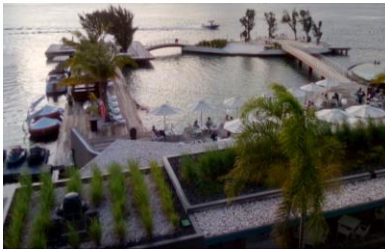
Green Roof (in foreground) Adjacent to Marina Source: Jacobs
