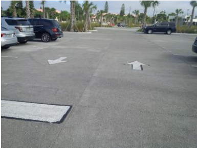
Pervious Concrete Parking Lot Source: Jacobs
