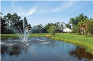
Wet Pond Source: Southwest Florida Water Management District
