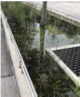
Stormwater Planter Source: Jacobs
