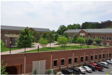
Blue-Green Roof Plaza Source: Jacobs
