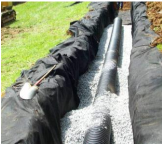
Infiltration Trench Source: Jacobs
